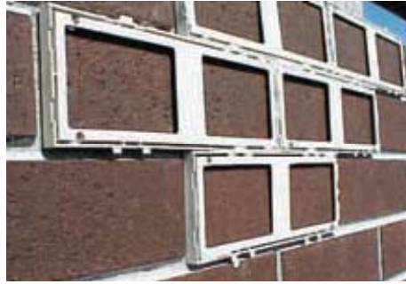
Templates Ready for Stripping
