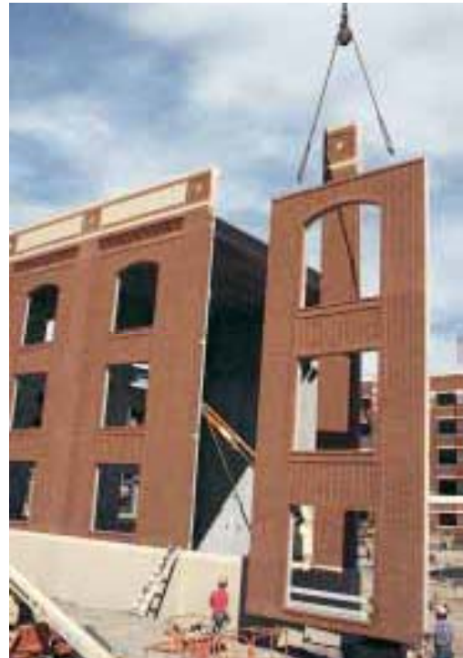
Panel Being Erected
