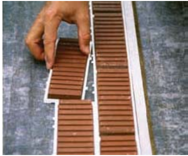
Thin Brick Being Laid in Form
